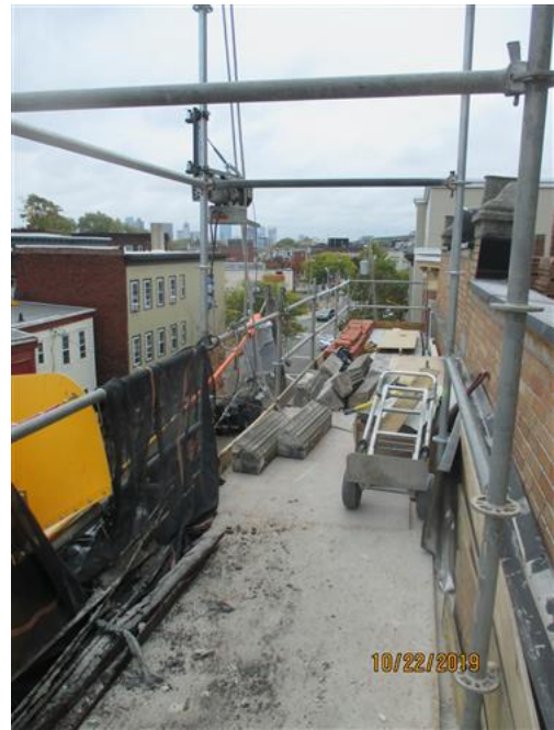
Chute and second hoisting area
