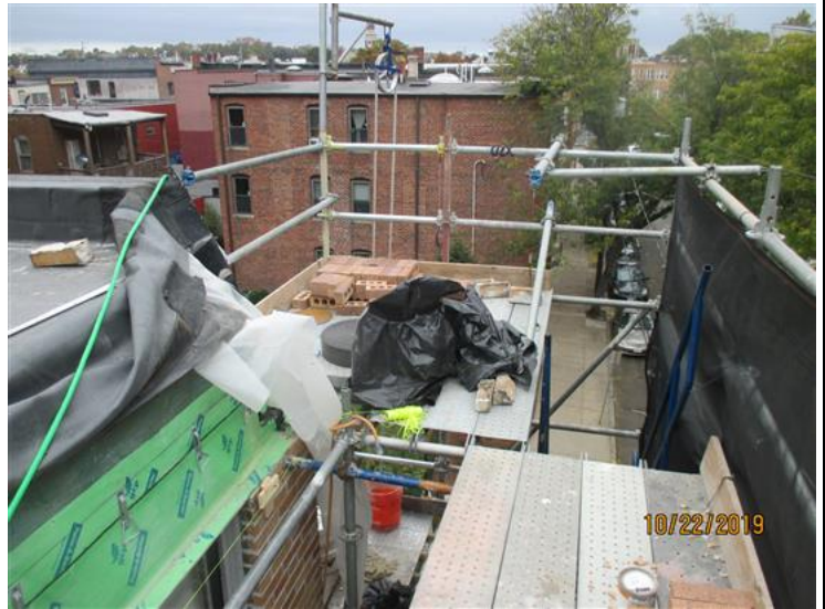
Hoisting area with open platform
