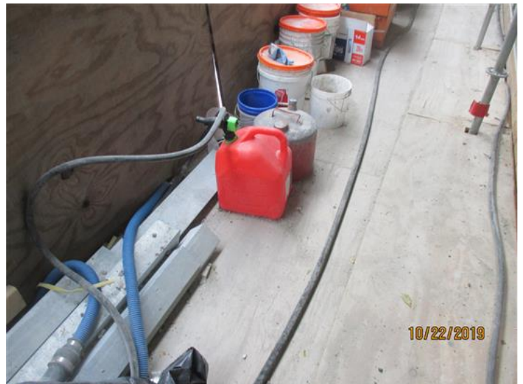
Improper Gas Can
